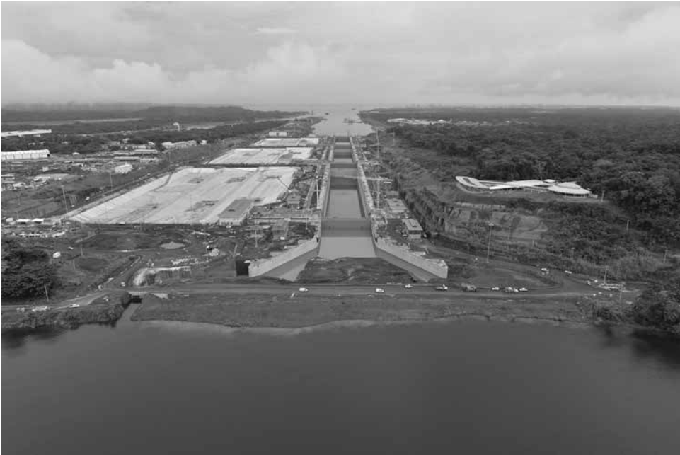
Figure 26.7 New Panama Canal locks under construction 2015
