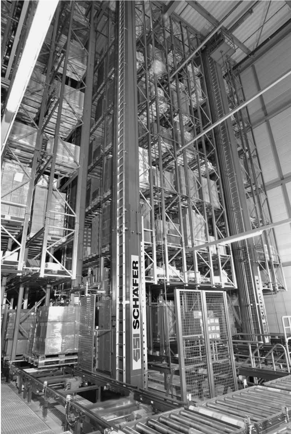
Figure 19.11 AS/RS crane, double-deep installation
