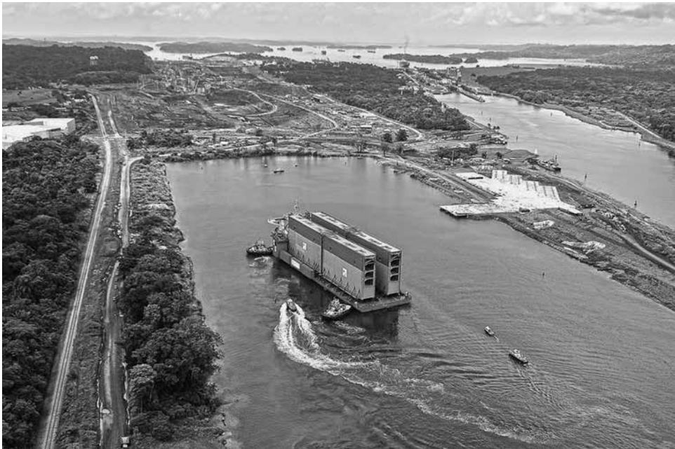
Figure 26.4 A heavy-lift ship delivering four new lock gates to the Panama Canal
