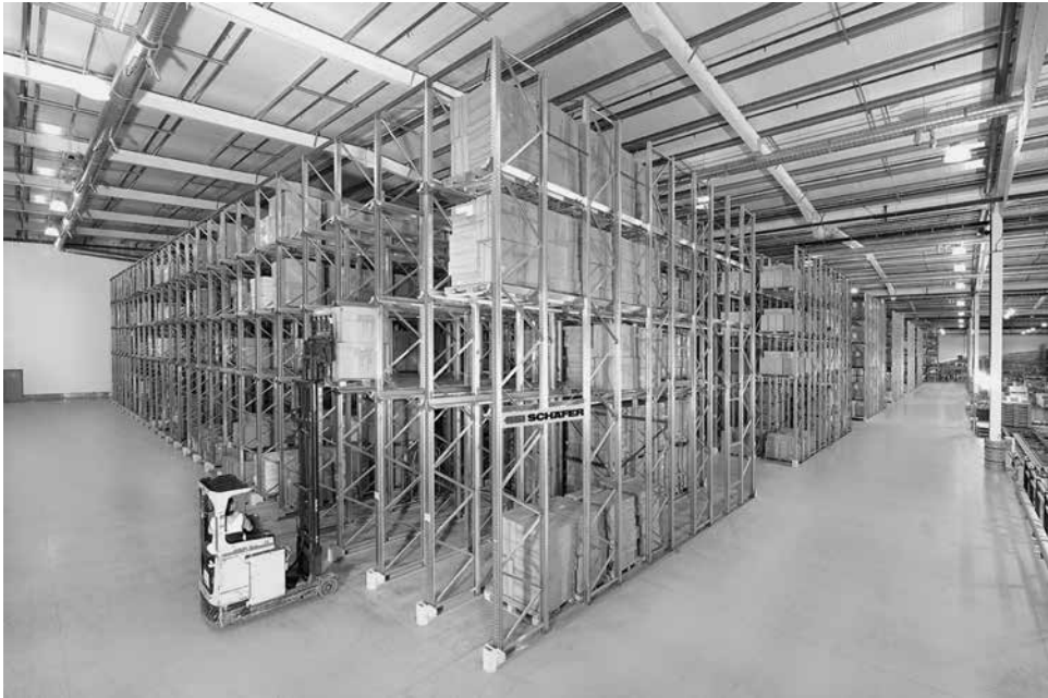
Figure 19.5 Drive-in racking being served by a reach truck
