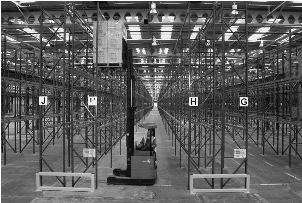
Figure 19.8 Newly constructed adjustable pallet racking being served by a reach truck
