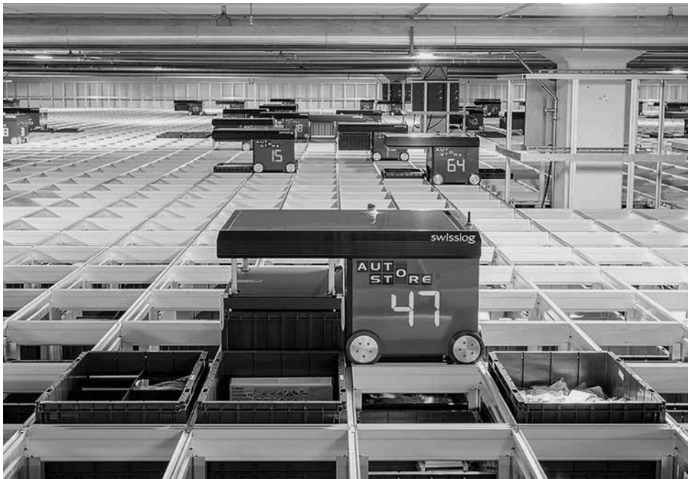
Figure 20.7 Multi-level grid system with robots extracting tote bins from the top
