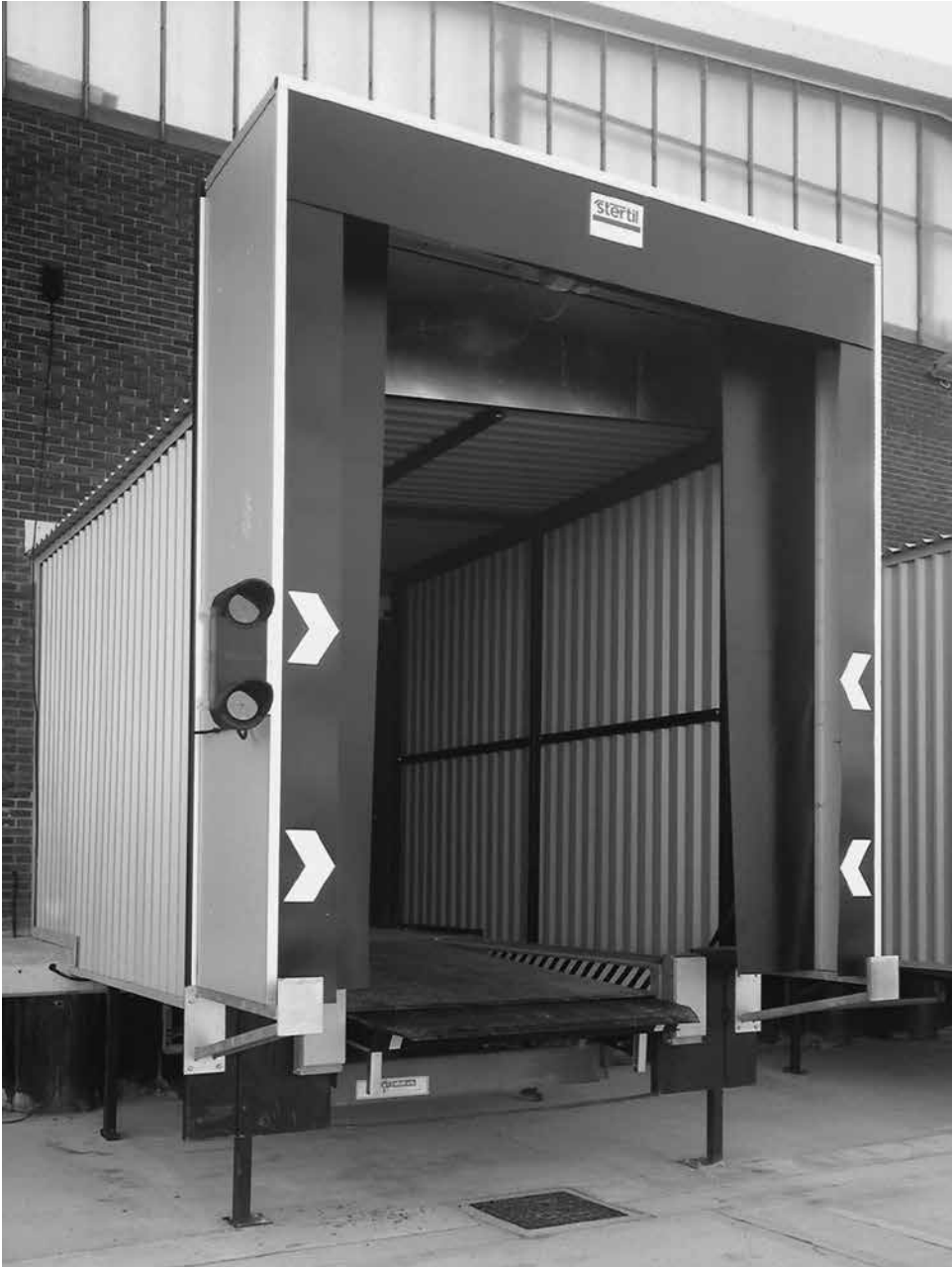
Figure 22.5 Dock house showing features such as seals, warning lights and dock leveller in a lowered position
